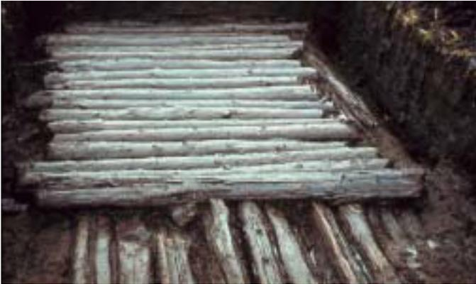
Fig. 23 The wooden pavement, *kavelbro*, of a medieval causeway, excavated close to a wetland in Trøndelag, Norway. (Photo: Ingrid Smedstad)
