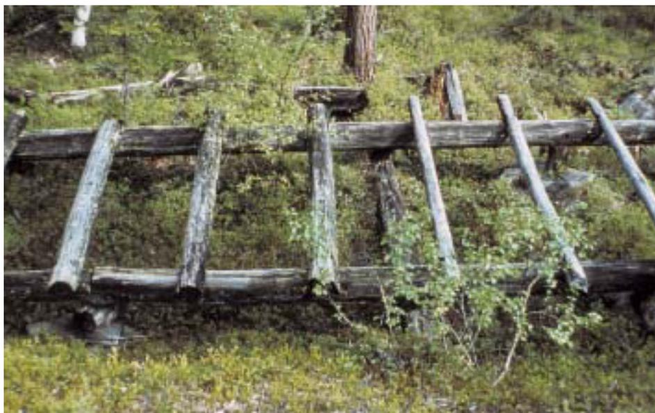
Fig. 13 Wooding hauling stand for boats used in timber floating along the Gargån River. This stretch of river consists of turbulent rapids and boats have to be dragged on land. This stand was originally built in 1909 and is still visible in the terrain. (Photo: Museum of Skellefteå in the 1970s)
